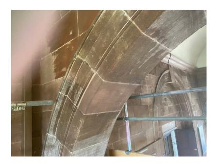
Good news that the repairs to the stone are now completed and hopefully the scaffolding will soon be removed. The photographs show the replacement stone and repair that has been carried out. The cornice is a plaster moulded section and the open joints have been patch pointed, the stone has been fixed using chem-set glue and a lime mortar mix for pointing any open joints. The new stone held itself in position due to the nature of the curve, and the glue was a secondary precaution only.
